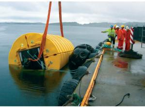
Modular Buoys can be used for mooring offshore vessels, compensating the weight of subsea structures and be included in the installation of subsea equipment.
